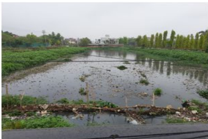
Drain flowing from west into the Beel
