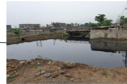
Drain entering from east through unauthorised colony
