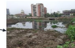
Drain Entering from South, showing silt deposition
