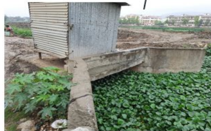
Drain Entering from South to the Beel
